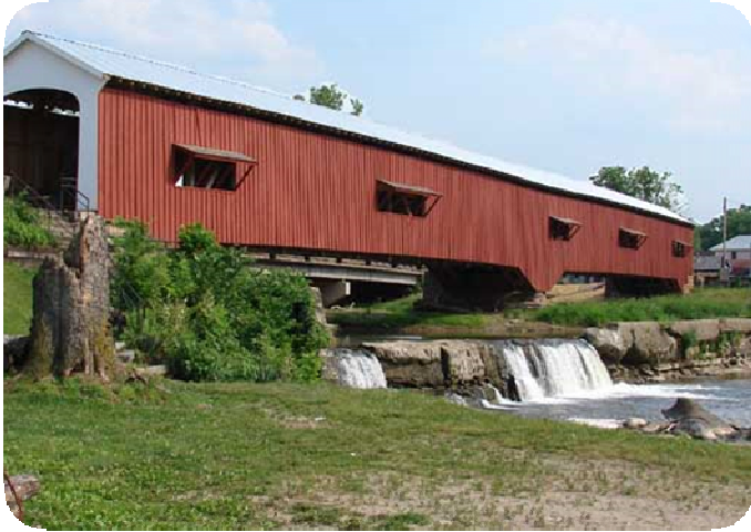
Bridgeton Covered Bridge
